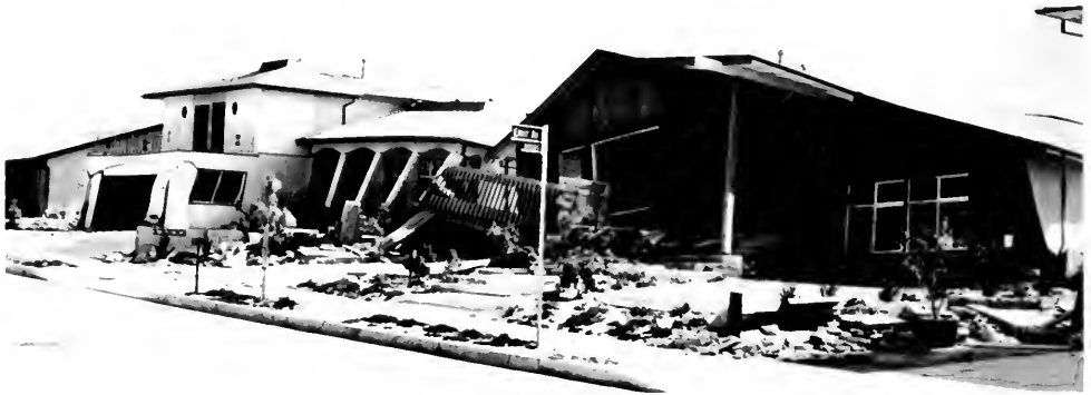
Photo 15. Examples of collapse of garage unit and support under single-story unit; house to left shown in photo 14.
